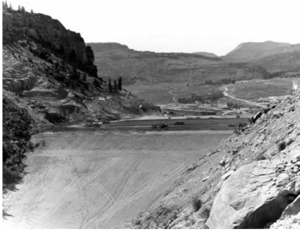
Photograph 6. Start of the embankment construction on Joes Valley Dam (1965).
